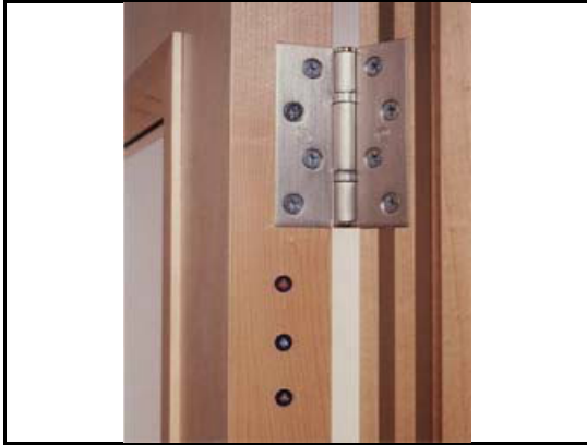
Image (above) fire rated hinge
