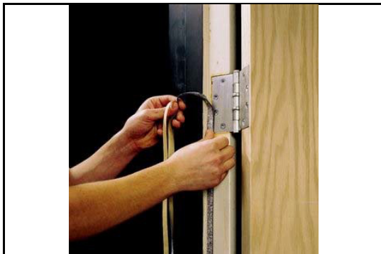
Image (above) shows smoke seal being fitted to a door frame
